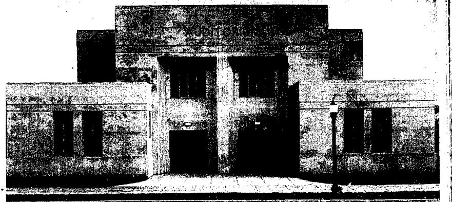
The Winside Auditorium was built in 1939 and took a year before it was completed. The building, still in use today,
